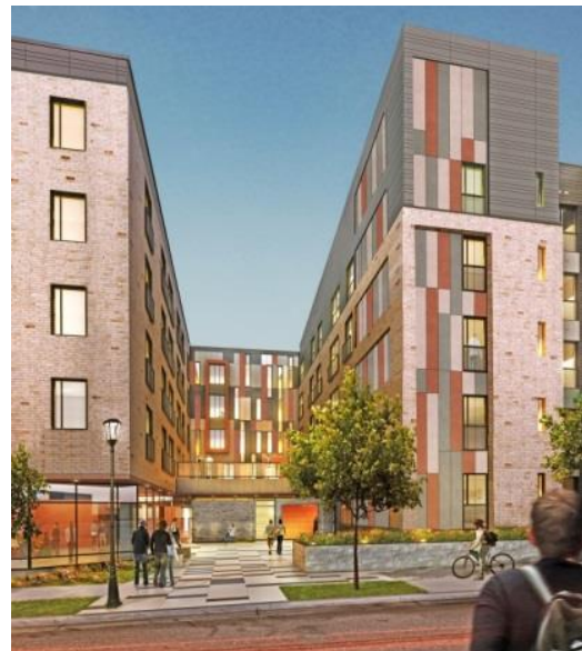
Courtyard fronting Thomas Street
